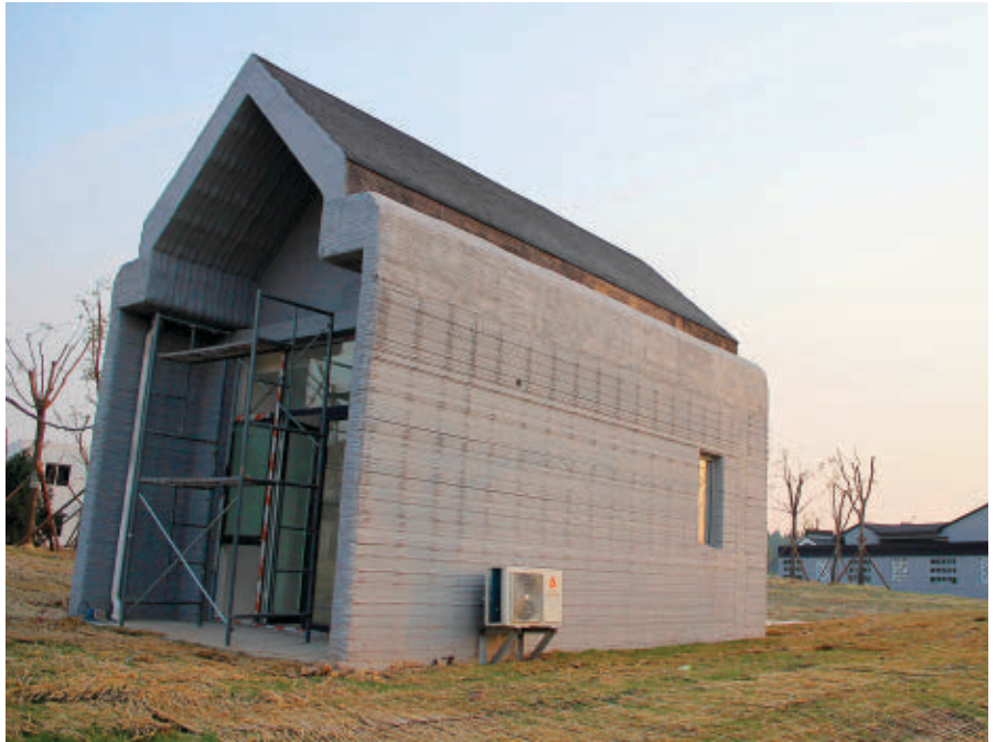
A concrete villa in Binzhou, China, that was produced by a 150-meter-tall 3D printer.
